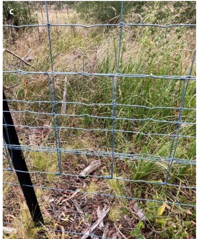
Figure 18. The partial sambar and fallow deer exclusion fence at Pheasant Creek Flora Reserve, North East Victoria: (a) a corner of the fence, (b) three-pin anchor (at gate post), (c) star post with raised apron, (d) double gate that can be opened to allow animals inside the fence to be mustered out, and (e) tree-fall over the fence requiring the tree to be cut up and the fence repaired
