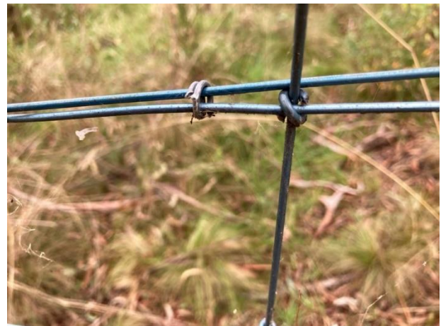
Figure 4. Prefabricated deer mesh netting clipped to a plain wire
