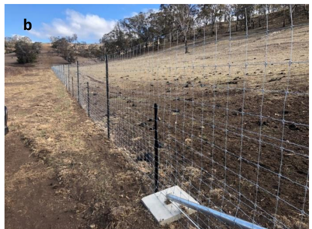
Figure 2. Two deer fence designs, both \geq 190 cm in height. (a) This design uses 190-cm-high netting with one high-tensile wire 15 cm above that and treated timber posts spaced at 5 m. (b) This design uses 190 cm-high netting (17/190/15) with steel star posts spaced at 5 m intervals (note alternating taller and shorter star posts).
