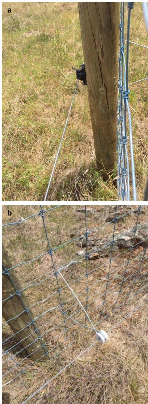
Figure 7. Examples of electric outriggers on (a) the inside and (b) the outside of a deer exclusion fence. Both outriggers are 50 cm above the ground, and the outside wire is 30 cm out from the fence. The objective of the inside outrigger is to prevent livestock (in this case sheep and cattle) from pressing against the fence. The outside outrigger prevents deer, macropods and livestock from pushing against the fence.
