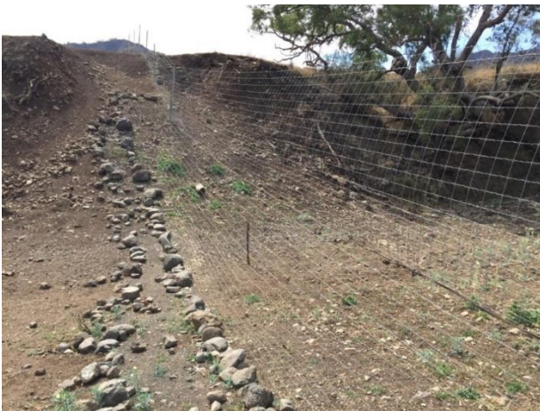
Figure 10. Exclusion fencing across a major creek that is expected to flood and destroy the lower section of netting. The steel cable holding the two sections of netting together can be seen most clearly in the lower right part of the image. A flood could be expected to remove the lower section of netting, which can easily be replaced. Note the large rocks holding the netting down across the dry creek bed.
