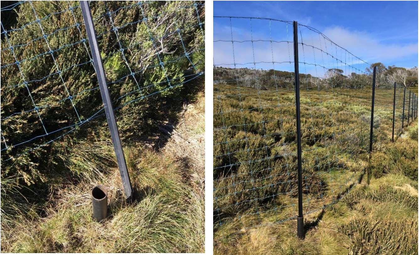
Figure 17. The drop-down section of the Maisie's Plot sambar deer and horse exclusion fence, Bogong High Plains, Victoria. This section of the fence is dropped prior to the first snows and erected when the snow has melted. Source: Elaine Thomas, Parks Victoria.
