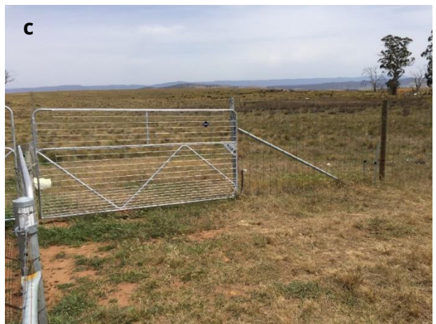
Figure 13. The Midlands, Tasmania, fence. Note the electric outriggers ('hotwires') inside and outside the fence 50 cm above ground level and (b) the 30 cm apron extending out from the fence.
