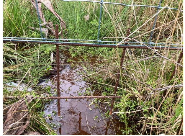
Figure 11. Concrete reinforcing mesh used to prevent deer and other animals from getting under a deer exclusion fence where it crosses a small creek.
