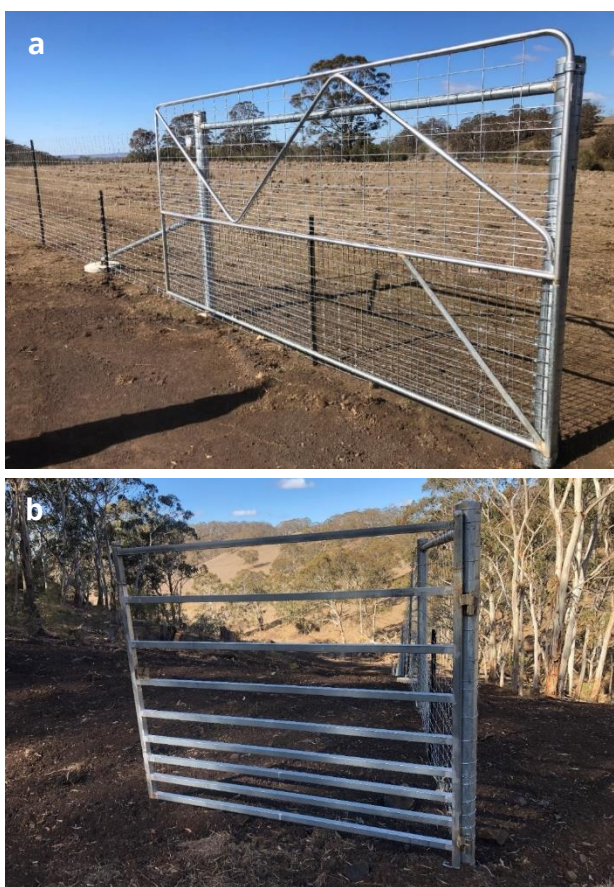
Figure 8. Two examples of gates for deer exclusion fences. In (a), two stock gates have been welded together and mesh welded to them (with smaller-size mesh on the lower part of the gate). In (b), the lower four rungs have been spaced at 10 cm intervals to prevent small deer from pushing through them.
