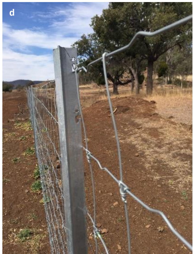
Figure 14. A Liverpool Plains, NSW, fence. Note the absence of plain wires (top, bottom and belly), rather, the mesh netting is tied directly to the posts and the apron is hinged.
