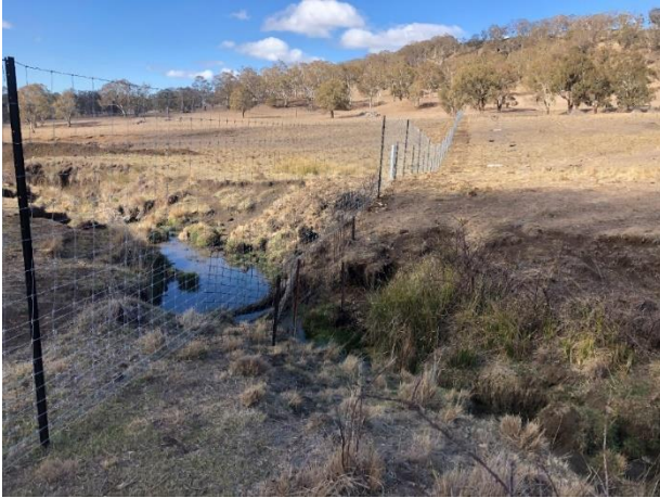
Figure 9. Exclusion fencing across a small creek that is not expected to flood frequently. The solid mesh is tied to star posts and to the deer fence.
