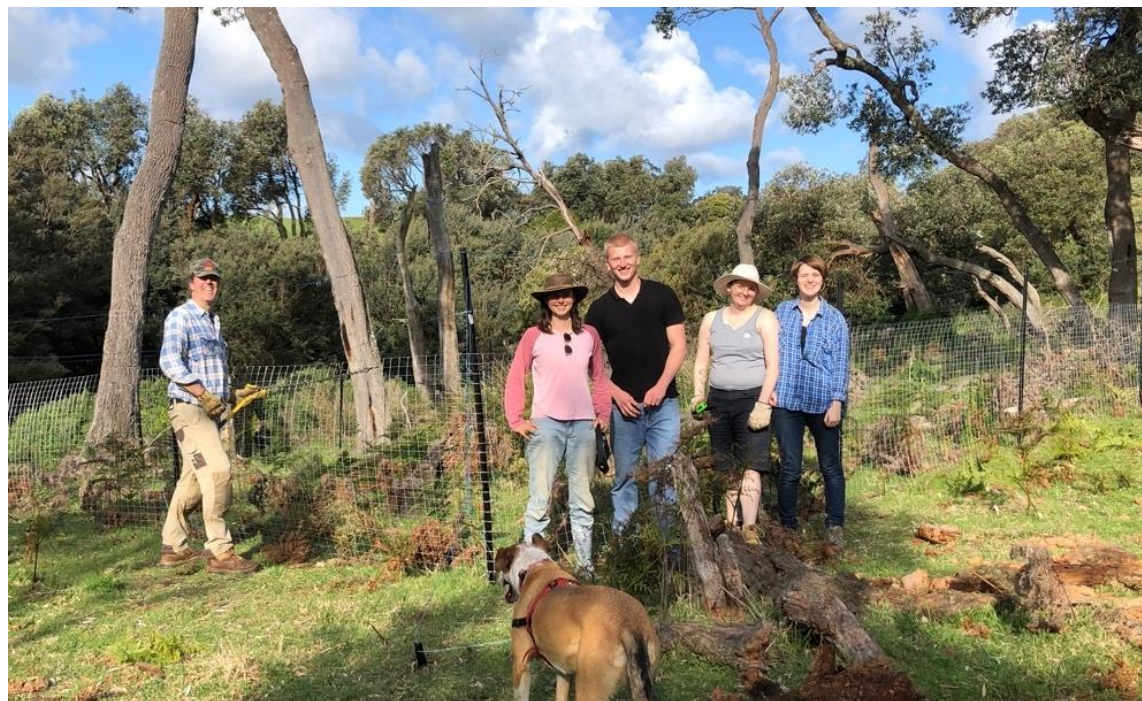
Figure 22. South Gippsland landholders installing fencing
